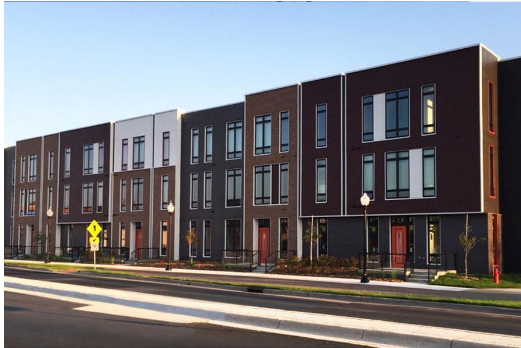
Artspace Hastings River Lofts, Hastings
